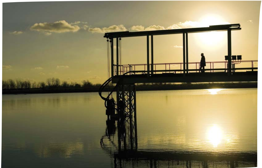
New compacting technology has been used to ensure that the life of the goethite residue ponds in Balen, Belgium, can be extended
