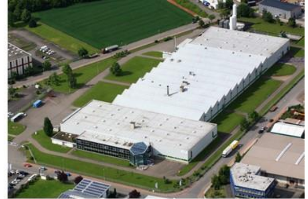
Bad-Säckingen plant AC, Germany
