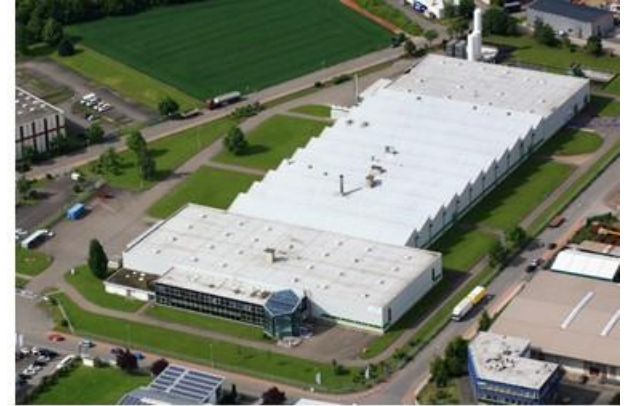
Bad-Säckingen plant AC, Germany
