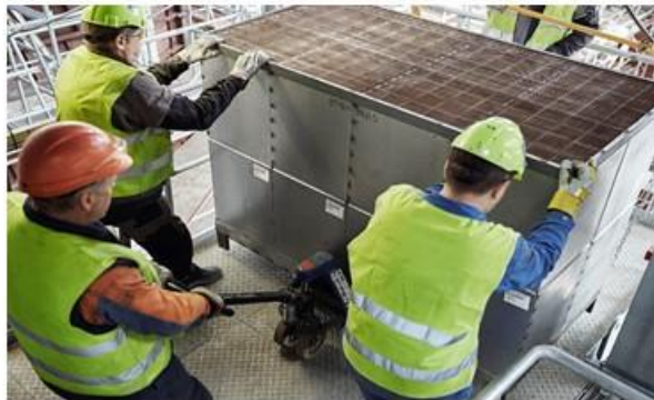
Installation stationary DNOx catalyst
