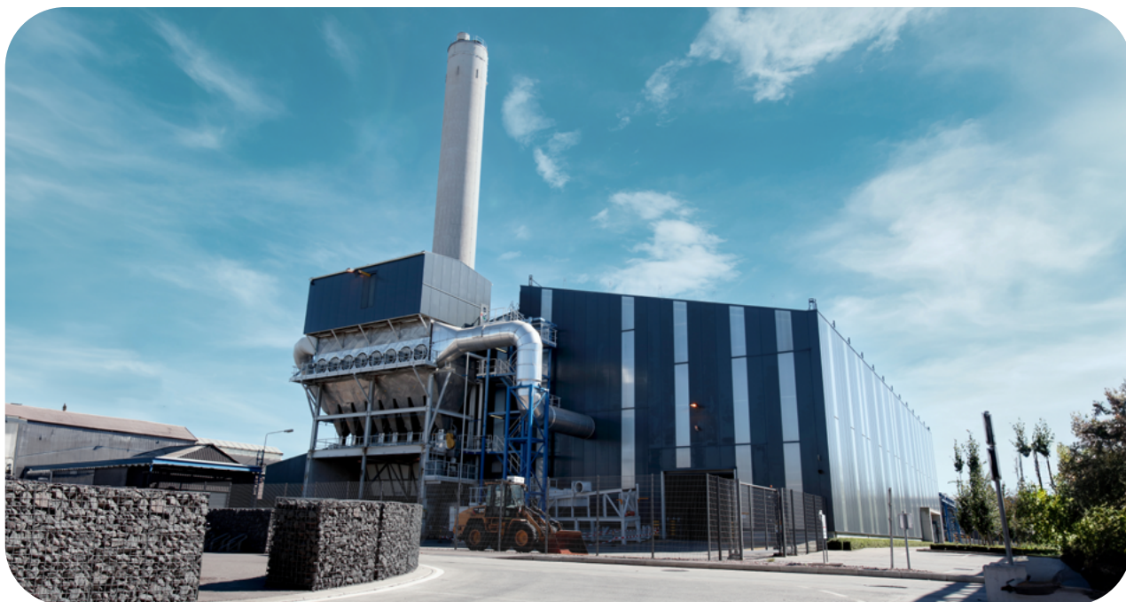
Umicore pilot battery recycling plant in Hoboken, Belgium.
