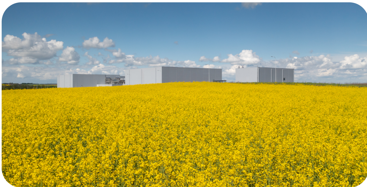
Umicore battery cathode materials plant in Nysa, Poland.
