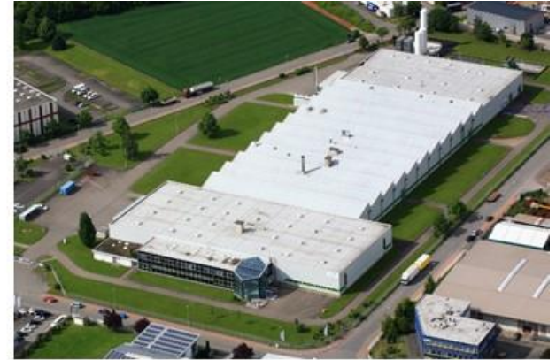
Bad-Säckingen plant AC, Germany
