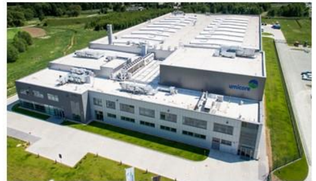
Nowa Ruda plant AC, Poland
