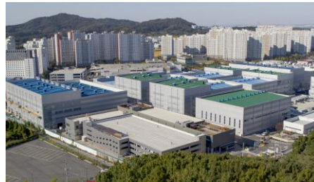
RBM cathode materials plant in Cheonan, Korea
